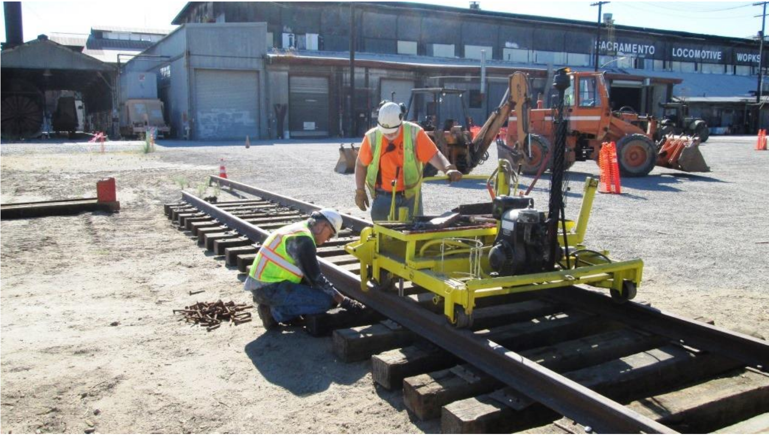
Frank operates the rail-lifter to lift the rail so that Steve can get tie-plate between its base and the tie
