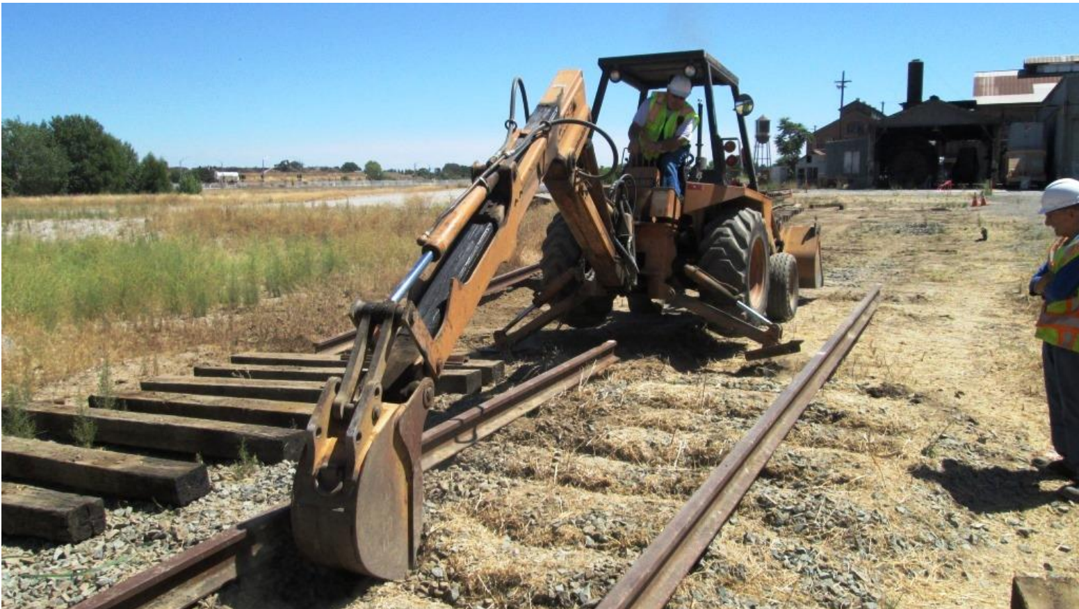
Harry V. starts digging away at the incredibly hard and compacted soil. The machine would lift up as the hoe tried to scrape the ground
