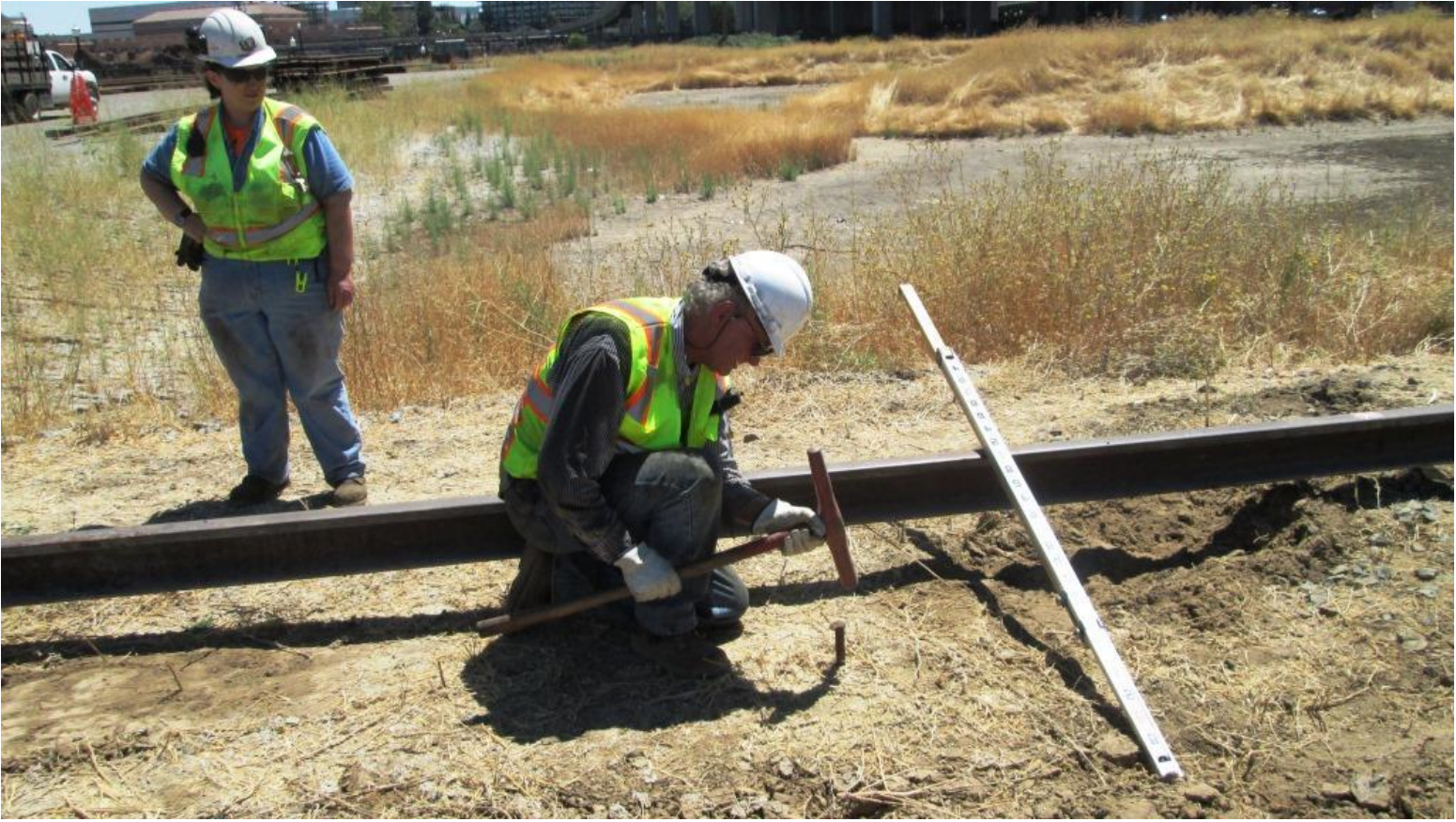
Steve drives a spike into the ground at the measured center-point of the track
