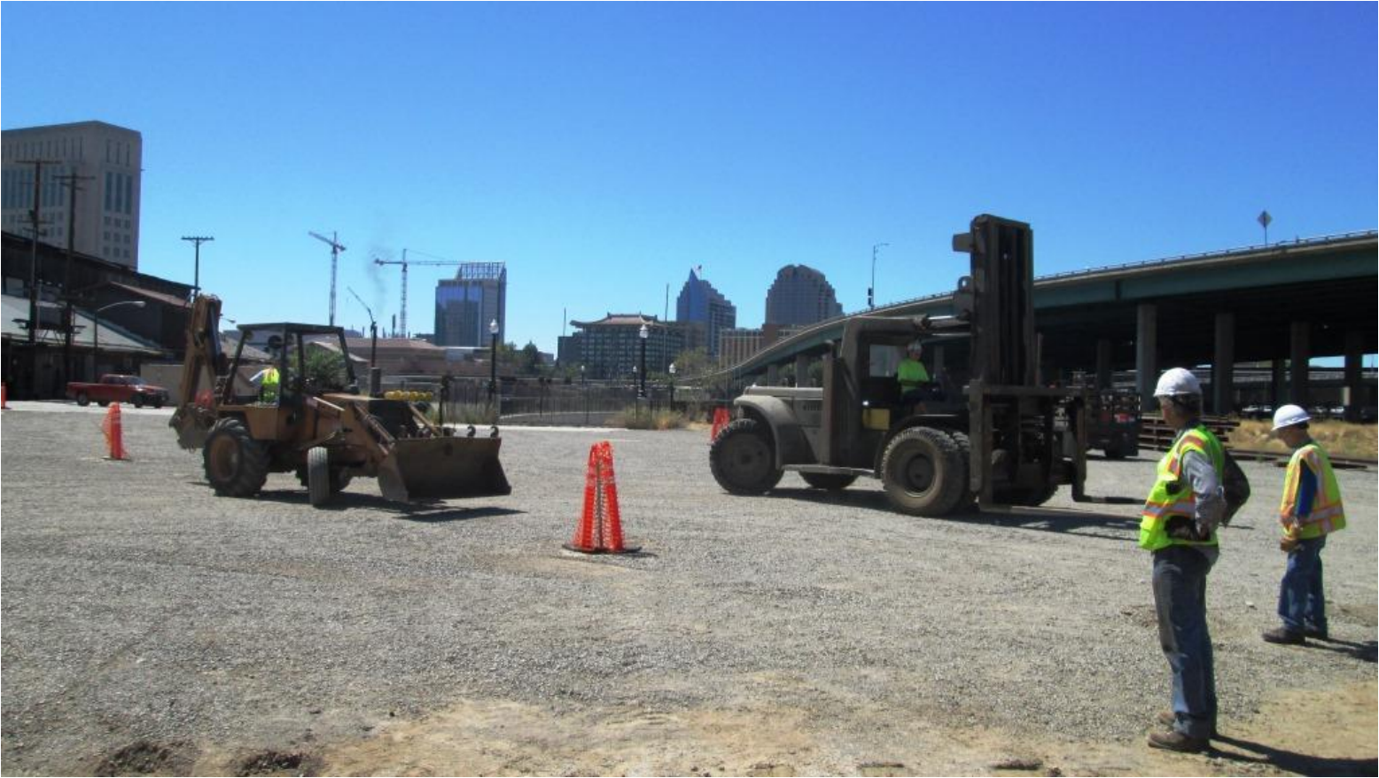
And now it's time for the big show. Harry V. on the back-hoe and Leonard on Simba get in position
