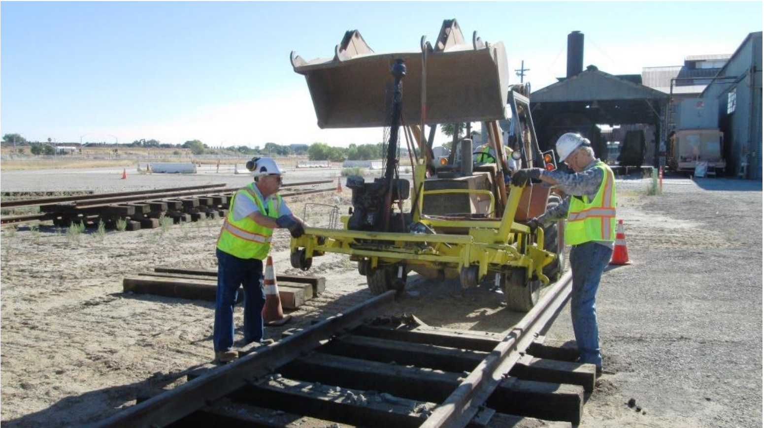
Clem and Oil-man Steve situated the rail-lifter on the rails
