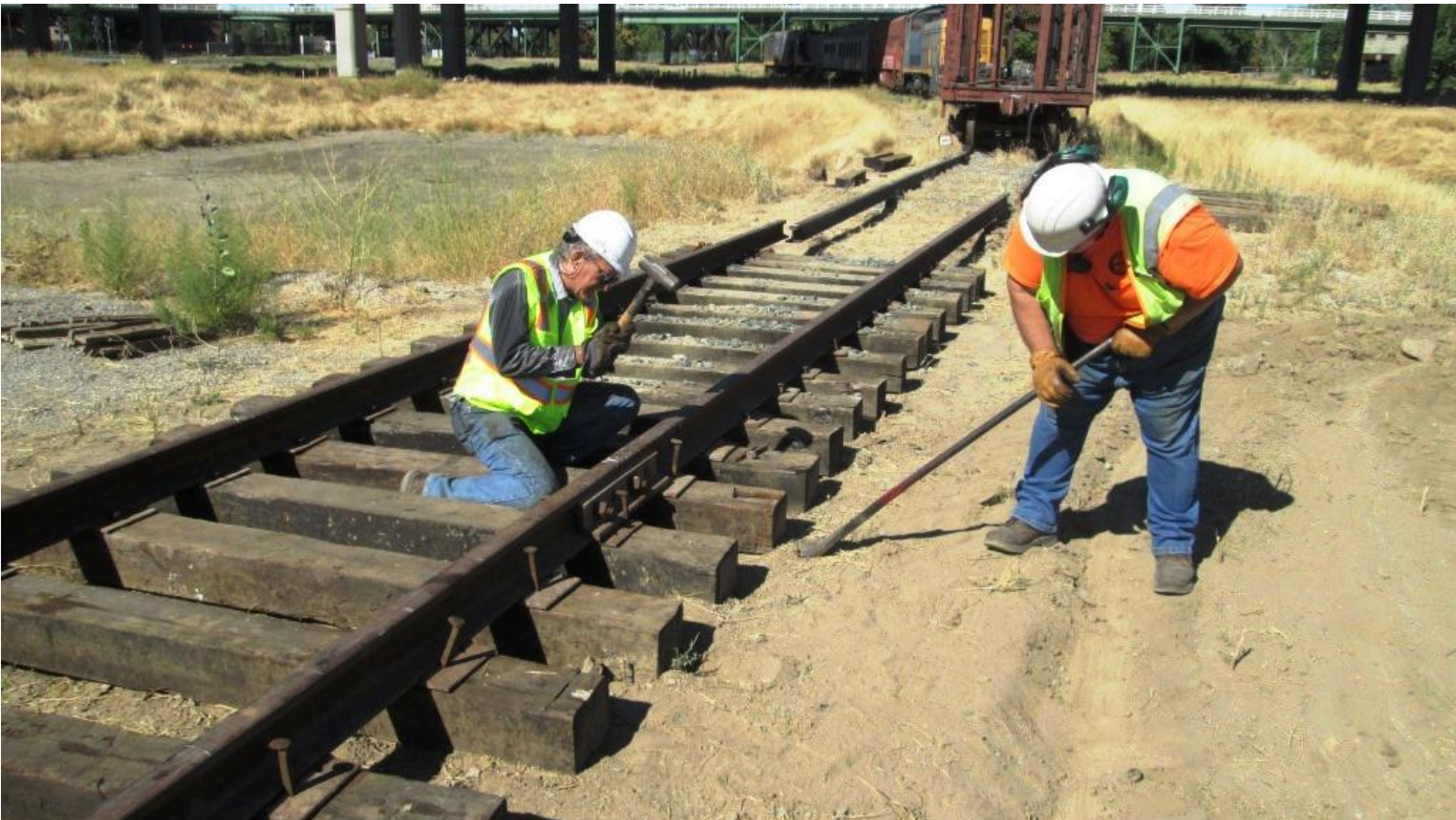
Frank nips-up the tie as Steve sets spikes. His shirt could be used as an oily-rag to fire-up the Granite Rock 10!
