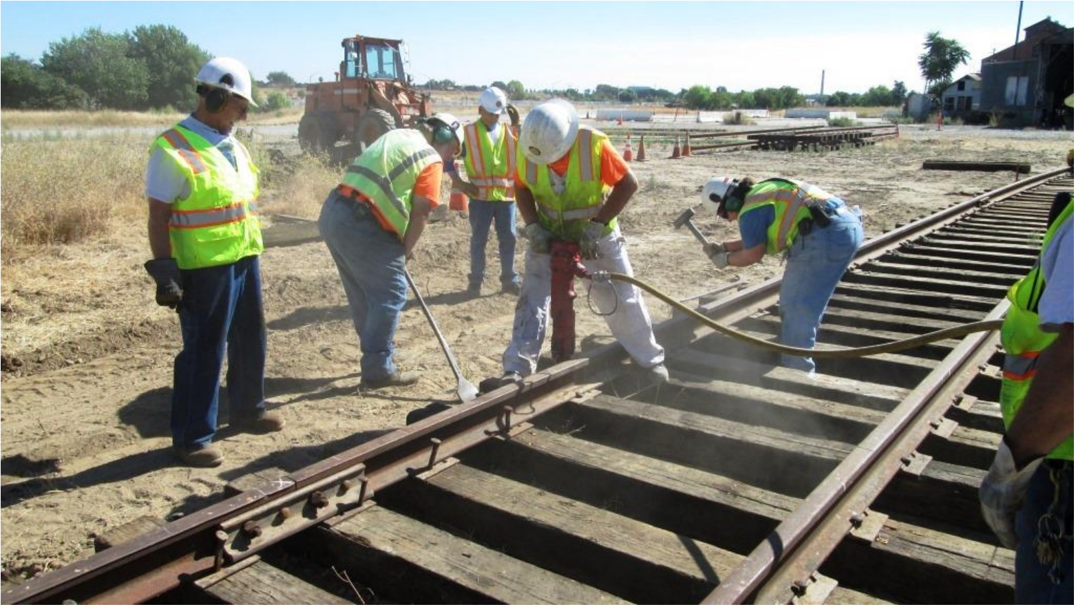
Driving spikes with the 60-pound spike driver is more fun than you can shake a stick and Mike did not want to miss out
