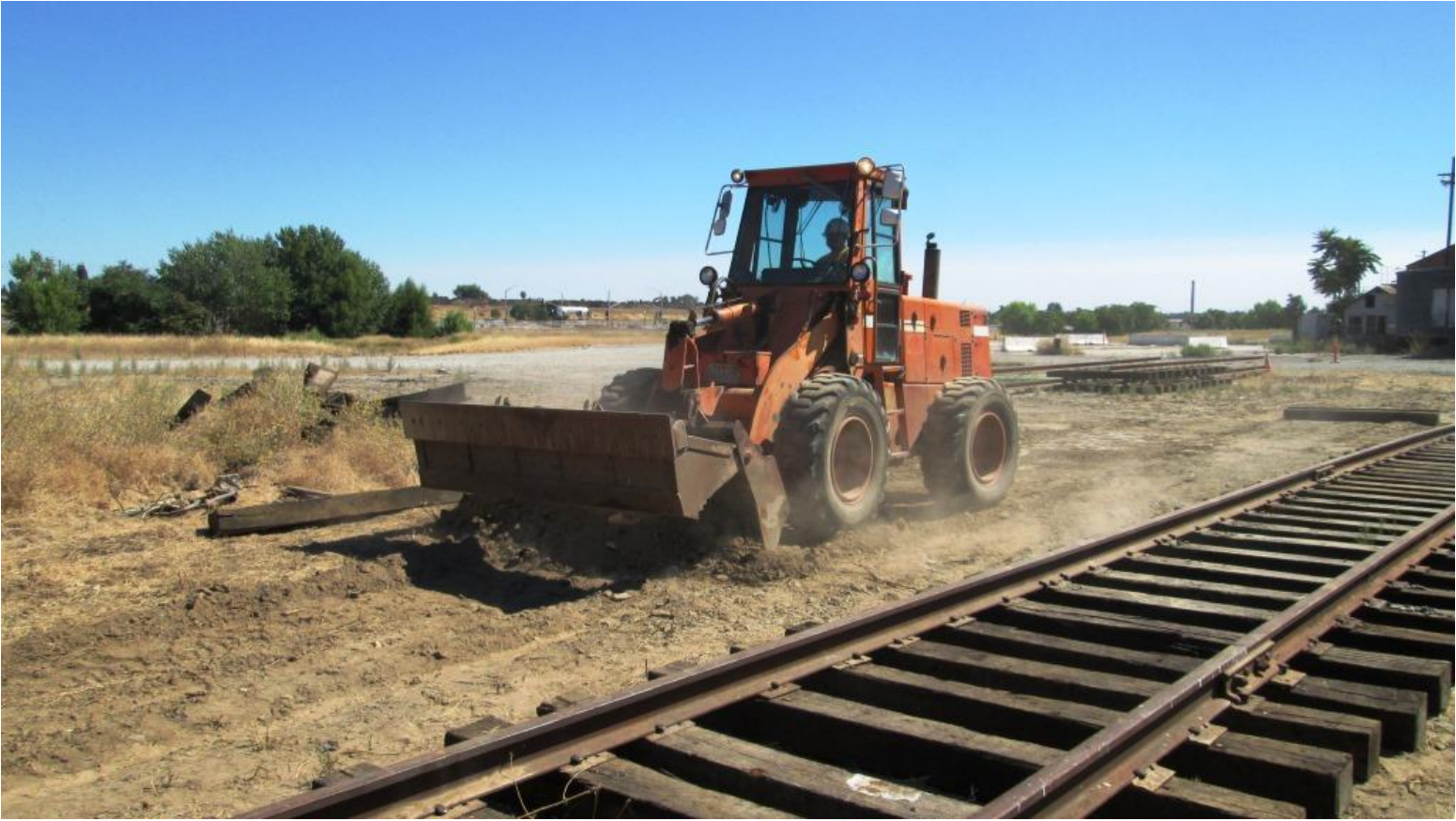
Mike uses the loader as a bulldozer to try to clear a path for the track as it moves north by about 11 feet
