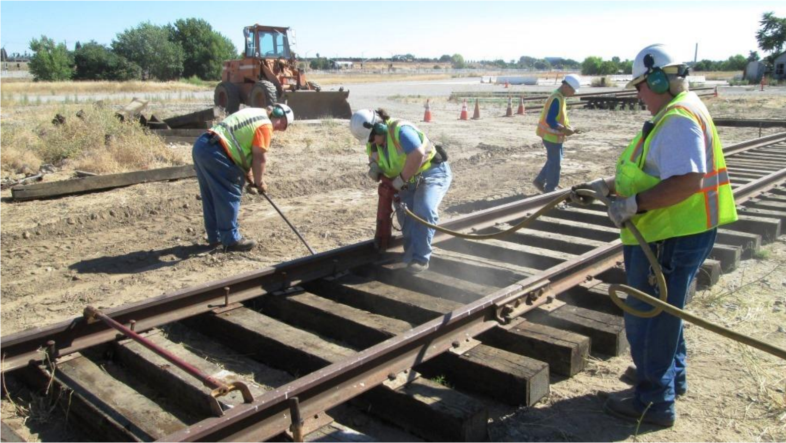
Heather is first-up on the pneumatic spike-driver. Frank nips-up the tie as Harry V. manages the air-hose
