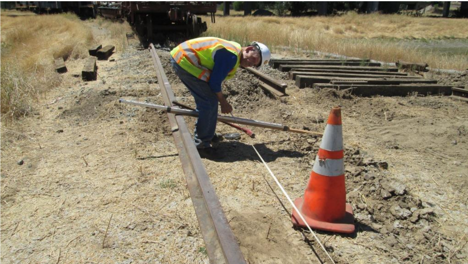
Harry G. measures and marks the centerline of the new track
