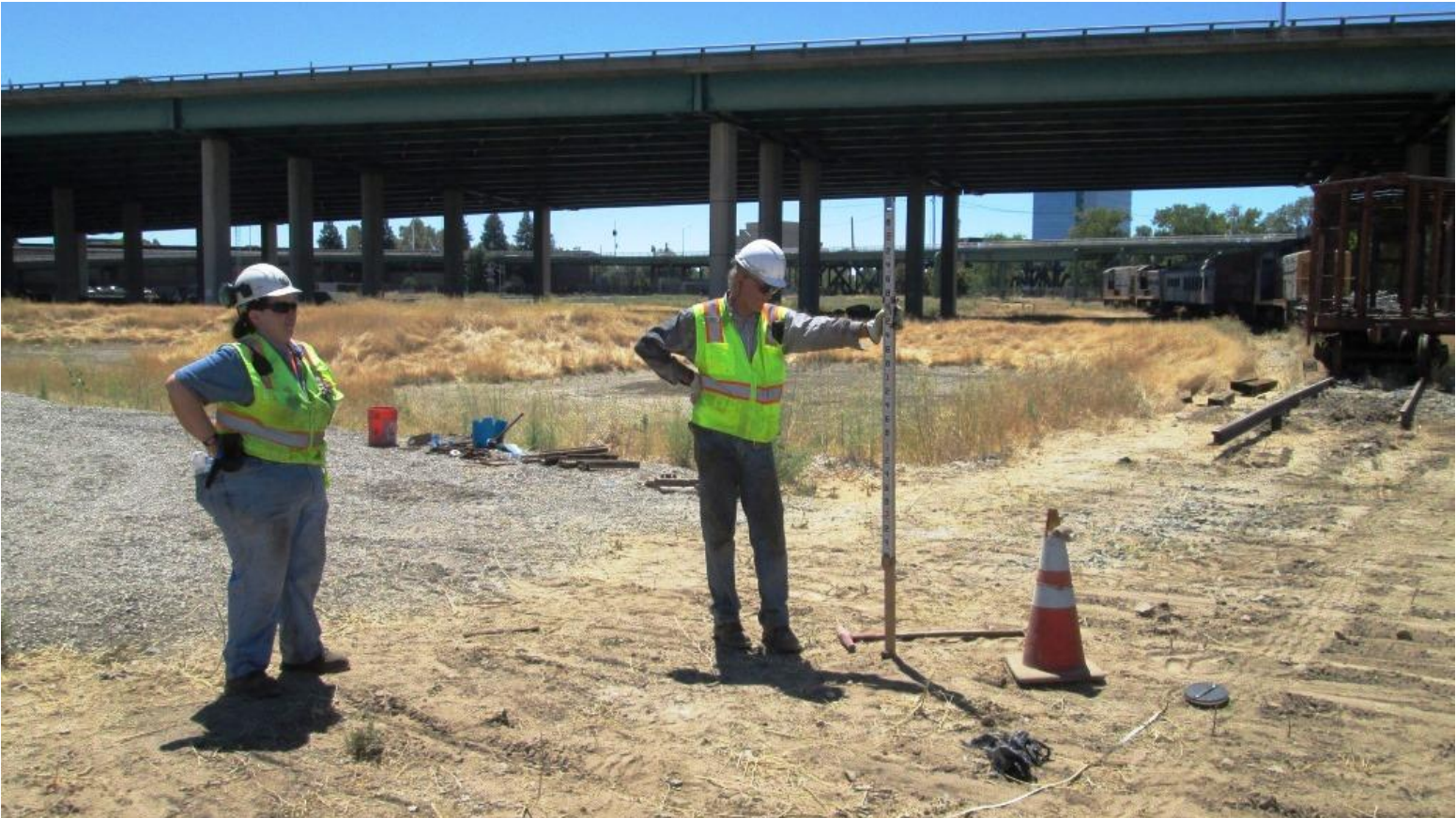
With the centerline marked, Heather and Steve place the measuring stick to Harry G. to sight the elevation
