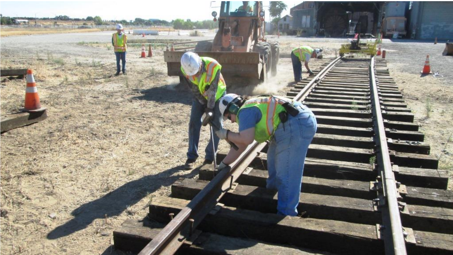
The Oil-man nips-up the tie as Heather sets spikes
