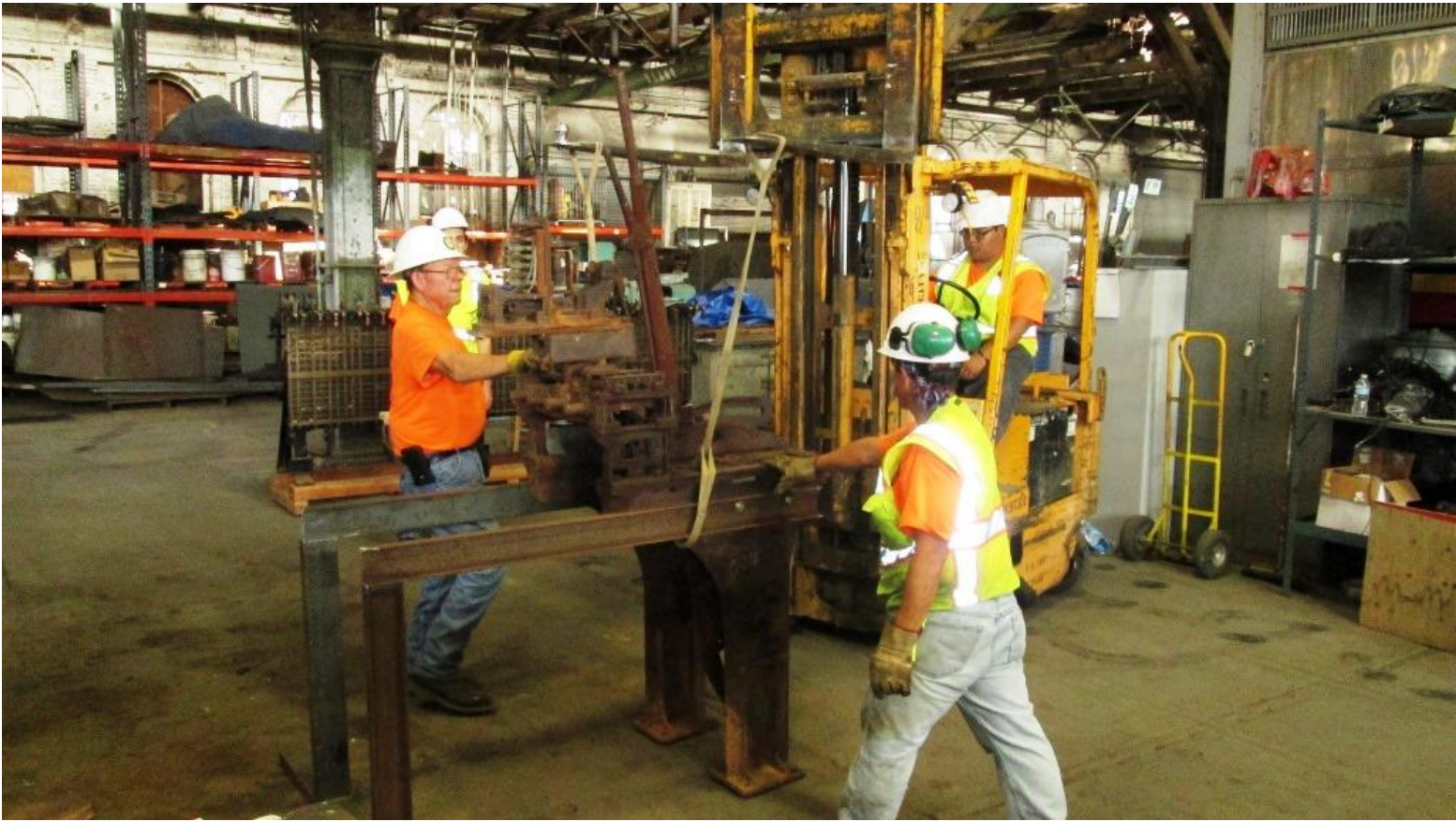
Cliff and Joe guide Anthony on the forklift as they relocate one of the switching devices that Team Signals is restoring
