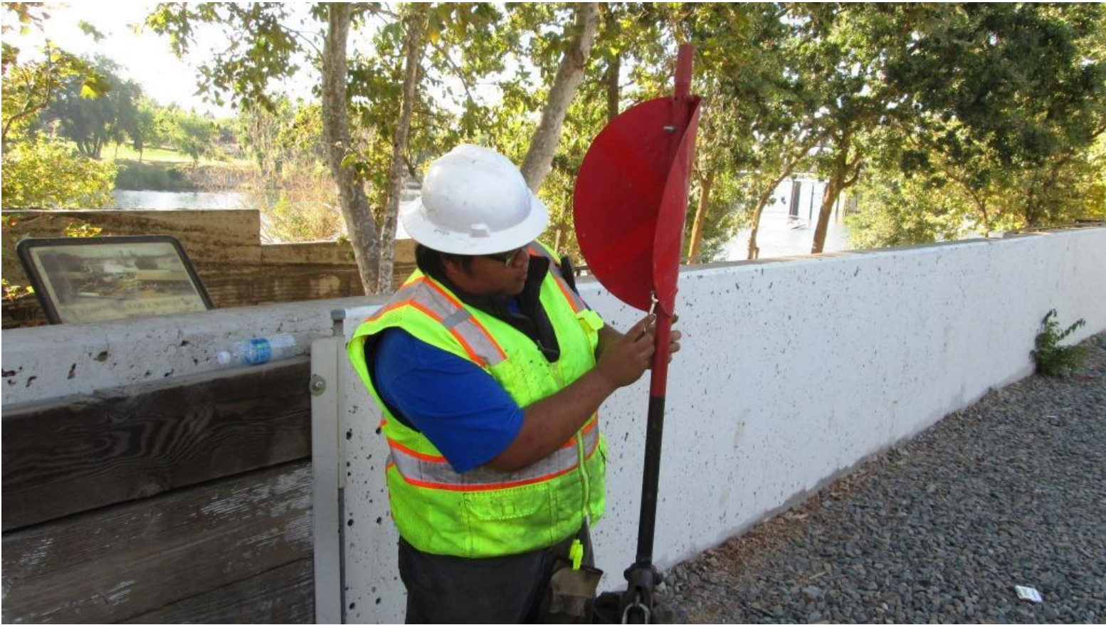
Anthony removing the pokey-damaged switch target on Switch 7
